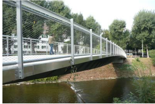
Fig. 6 Stückisteg footbridge, Basel, Switzerland.
