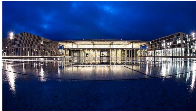
The terminal building at the construction site of the new 'Willy Brandt' Berlin Brandenburg International (BER) airport. The new airport has been plagued with problems, undermining Germany's reputation for engineering skill. Photo: Bloomberg
