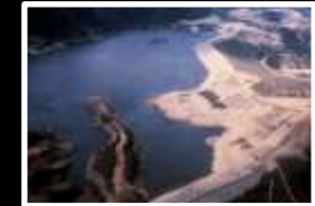
26. HIDROELECTRICA SAN CARLOS COLOMBIA
