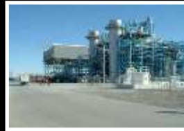
43. TERMoeLECTRICA SAMALAYUCA II
