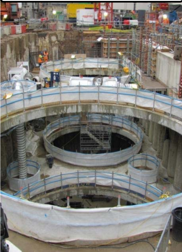
Bond Street East Ticket Hall
